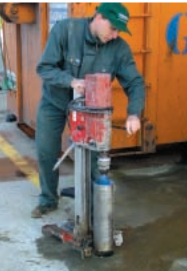
Soil sample being taken from underneath a concrete slab.
