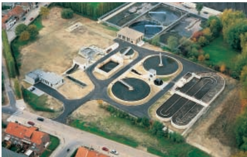
At Schoten WWTP the standards were no longer exceeded after the influent screw pumps were covered.
