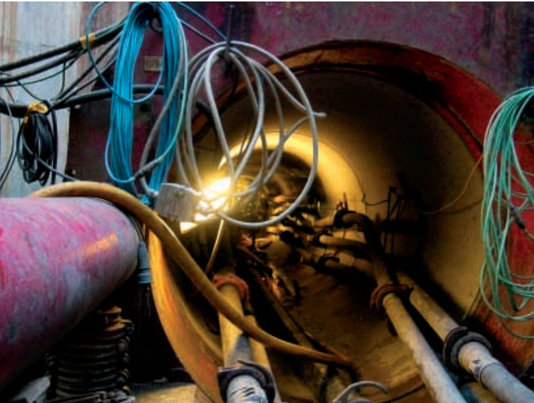
Thrustboring of a trunk sewer under the river Dijle in Mechelen.
