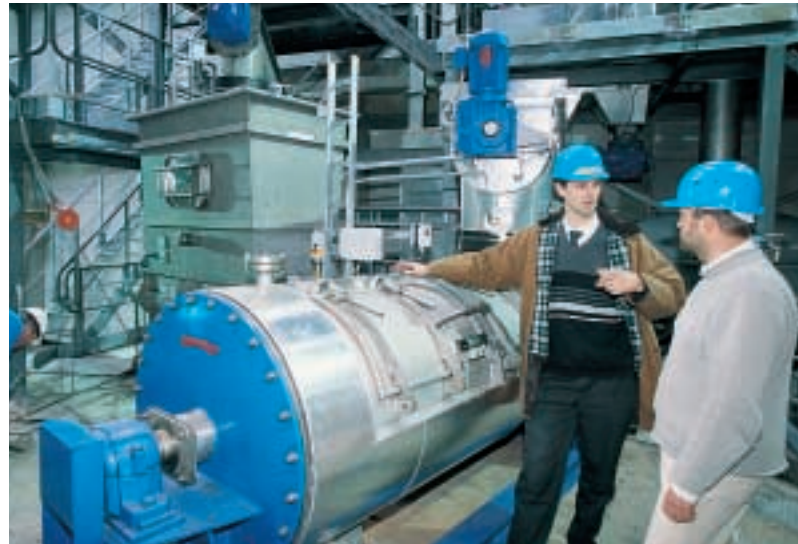
The new dryer on top of the sludge incinerator in Bruges.
