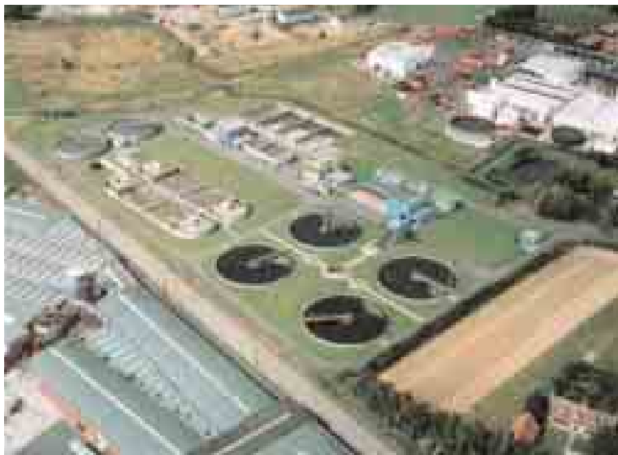
Roeselare wastewater treatment plant.
