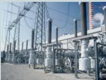
Transmission and distribution of Power 输配电
